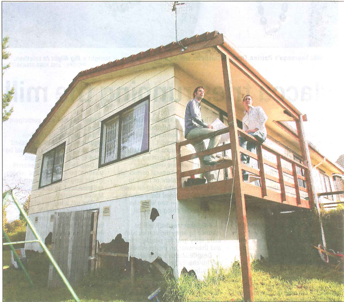
MAKE UP: The Makeover Project — Merivale project leader Joel Milgate (right) and head of the construction team Brian Miller at the makeover house in Hampton Terrace.
